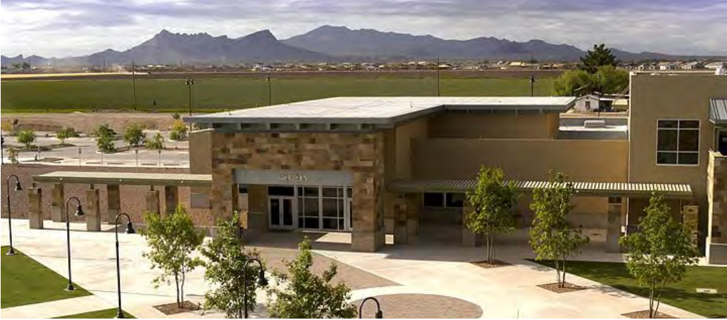
Municipal Complex in Northwest Marana; Photo: Kelly, Wright & Associates, PC
